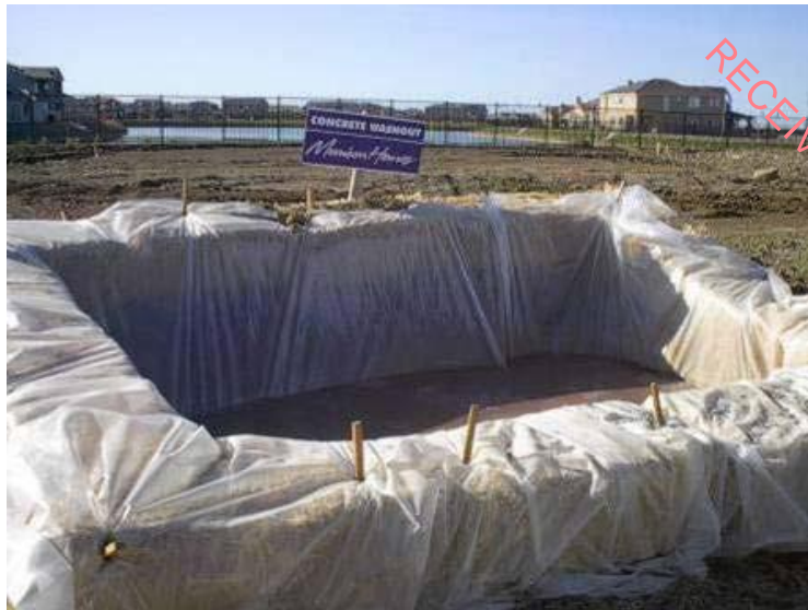
Plate 2.1: Typical Temporary Concrete Washout Area
